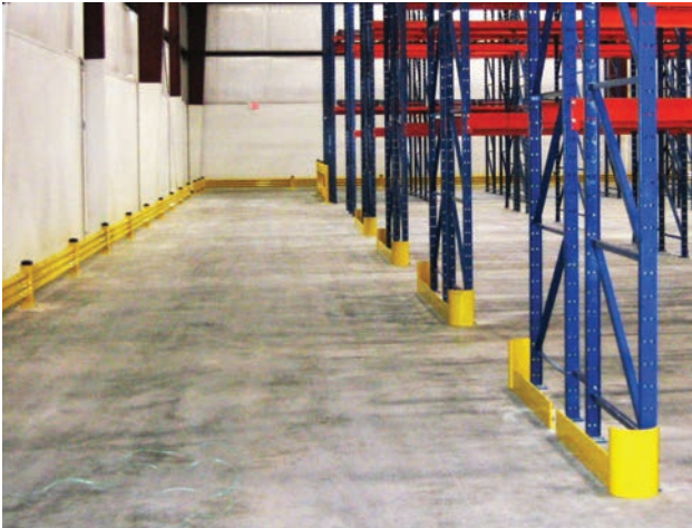
Perimeter protection and rack guard
